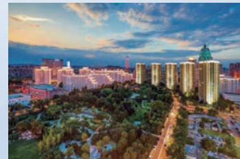
Exterior view of North Star Hui Yuan Apartment
