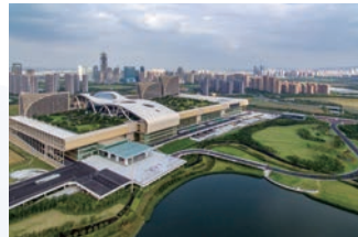
Exterior view of Hangzhou International Expo Center
