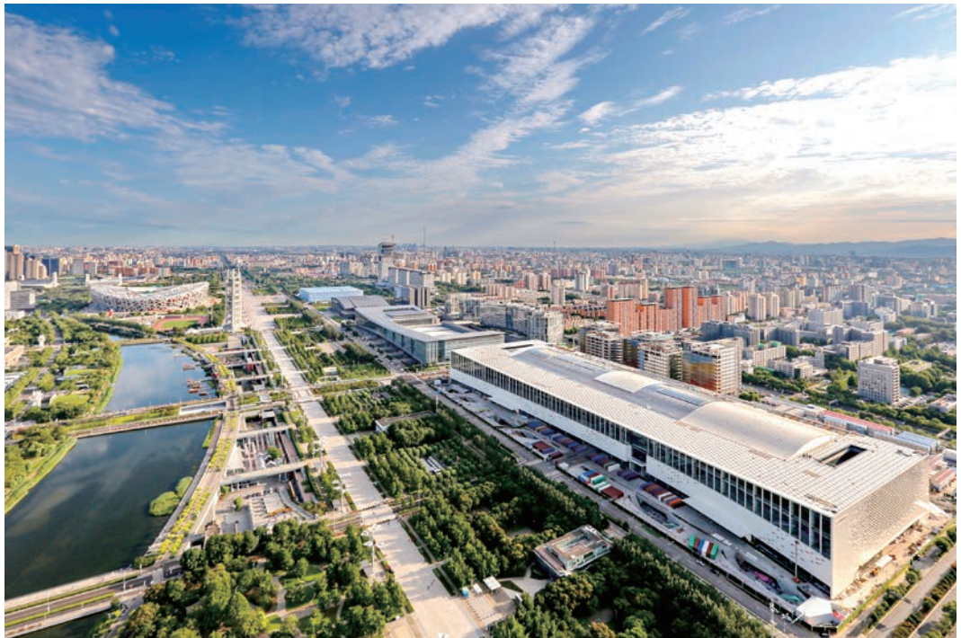
Main Media Center for the Winter Olympics
